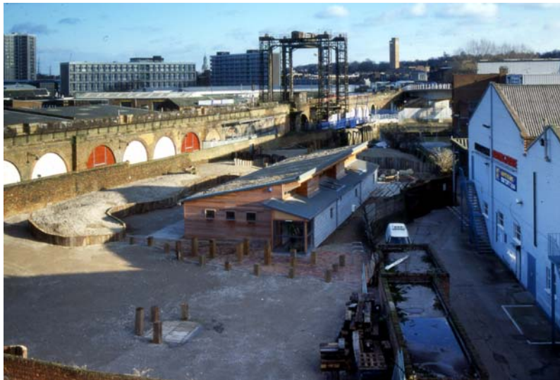
Aerial view of building within overall site
