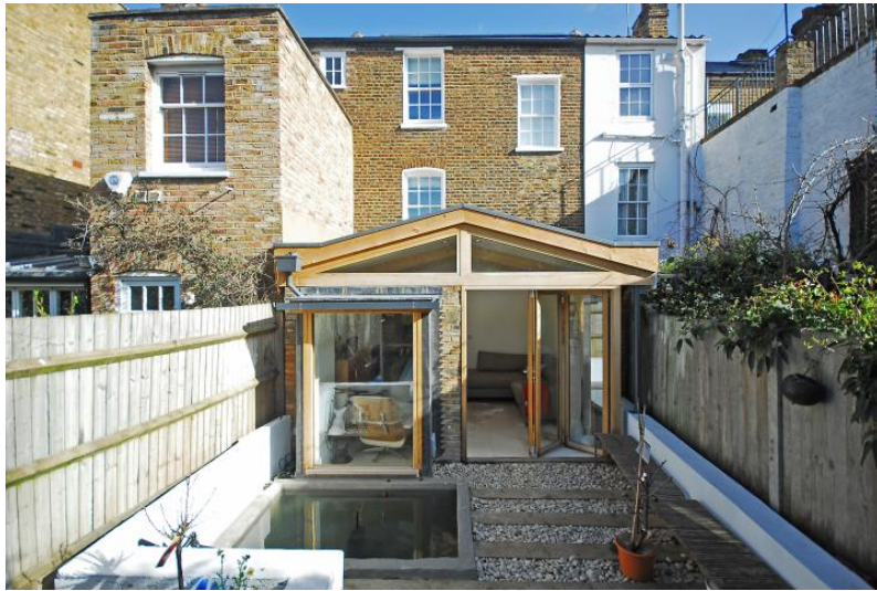
Rear elevation showing nature of extension
